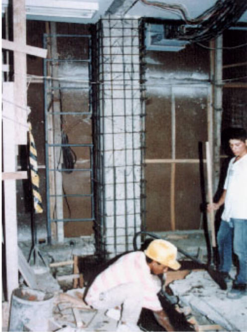
New added longitudinal and transversal reinforcement.
