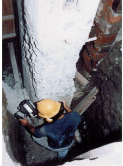
Anchorage of the new longitudinal reinforcement into the foundation
