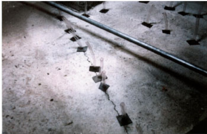
Epoxy injection of the cracks
