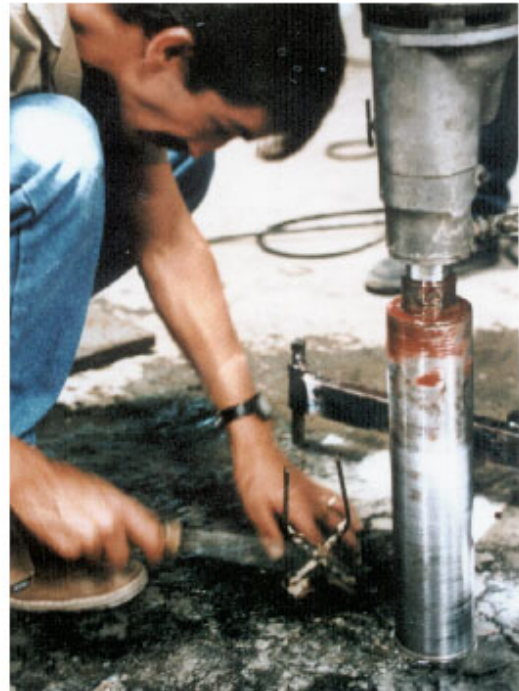
Extraction of concrete cores
