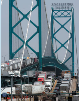
The Ambassador bridge connects Detroit in the United States to Windsor in Canada. On a typical day, $250 million worth of cars and car parts crosses this bridge.
