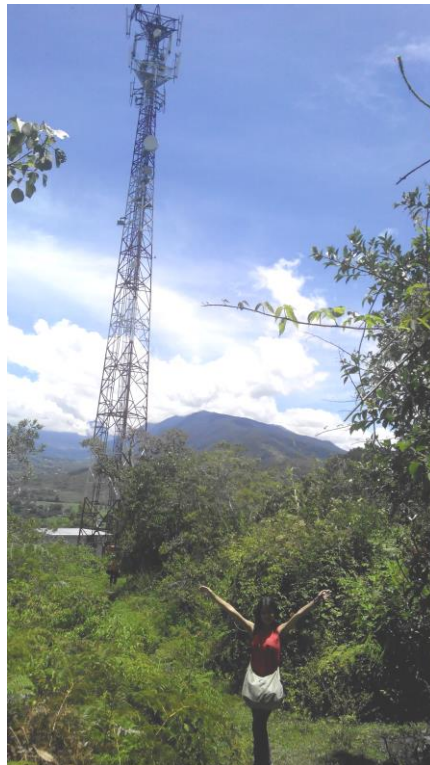
Figura 31 Radio Base de 48 mts. Loma Mucujun. Movinet
