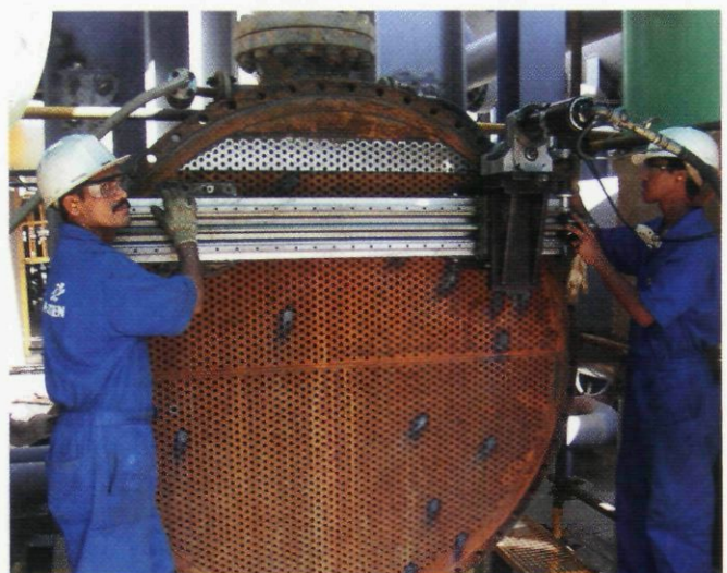
FIG. 5 In situ machining of the exchanger TTSJs.
