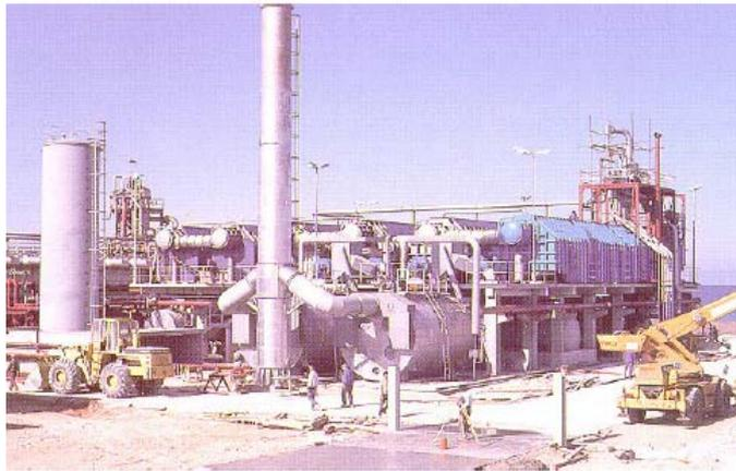
**MSF once-through long-tube evaporation plant
